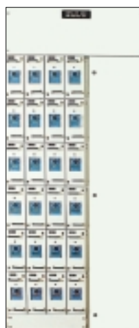
Inner view of motor control center type H8PU-S7
